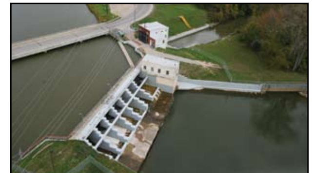
Beaverton Hydroelectric Dam
