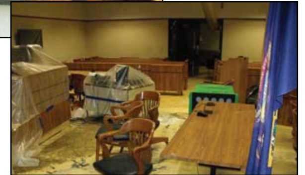
The restoration project, including this courtroom, required the replacement of drywall, carpet, and millwork damaged by the flood.
