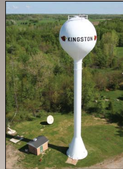
Kingston Water Tower
